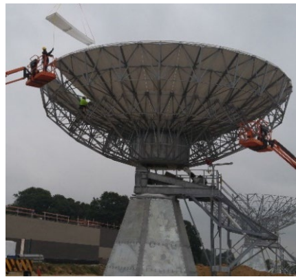
The installation by TSS Solutions included mechanical assembly and leveling of the pedestal mount.
